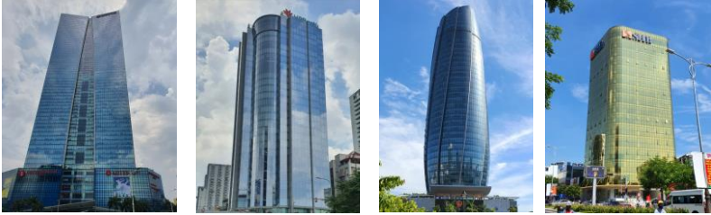
Figure 2.3. Typical examples of modern high-rise buildings in Vietnam use glass in a very large proportion on the facade (Lotte Hanoi, VP Bank Hanoi, TTHC Da Nang and SHB Da Nang).
